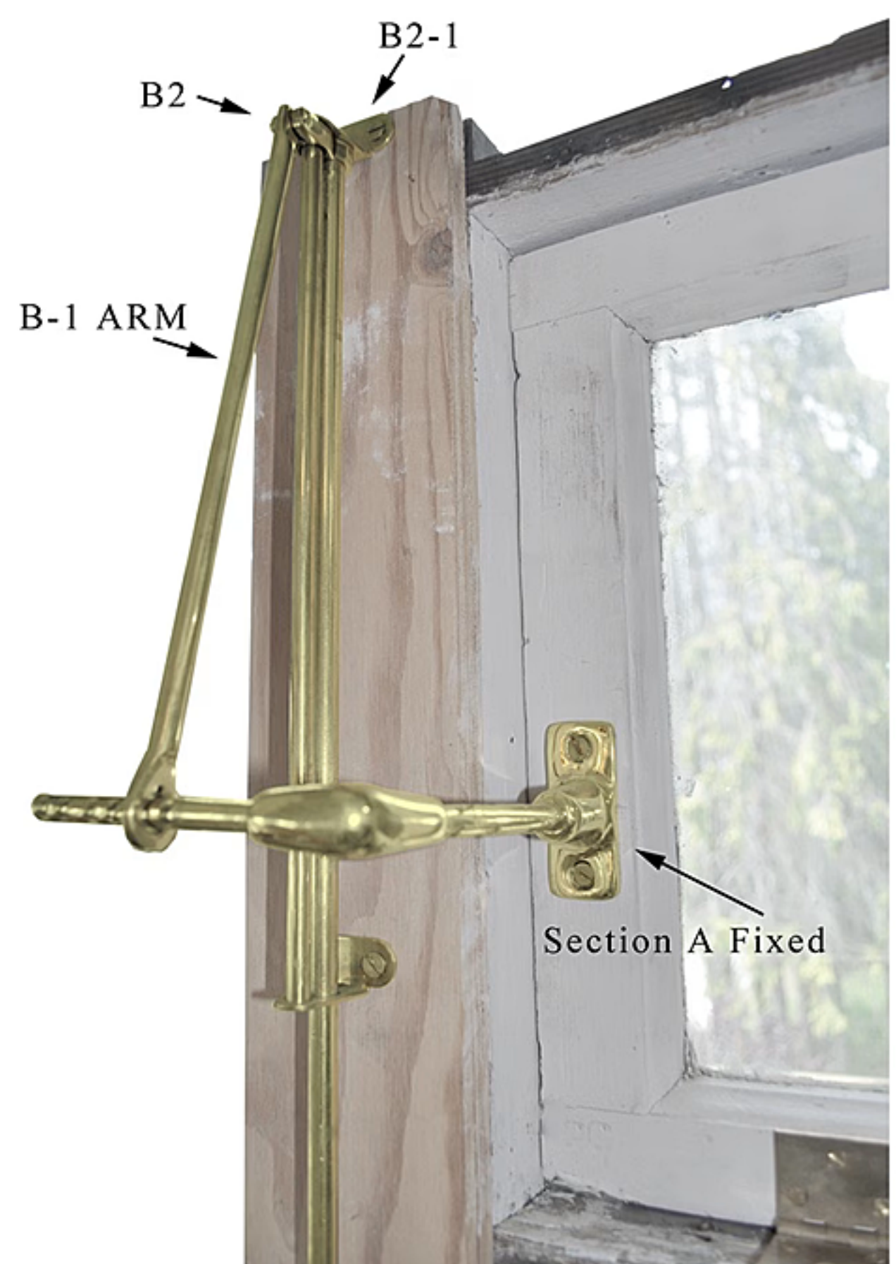
Placing Section "B" into Position with Section "A"
